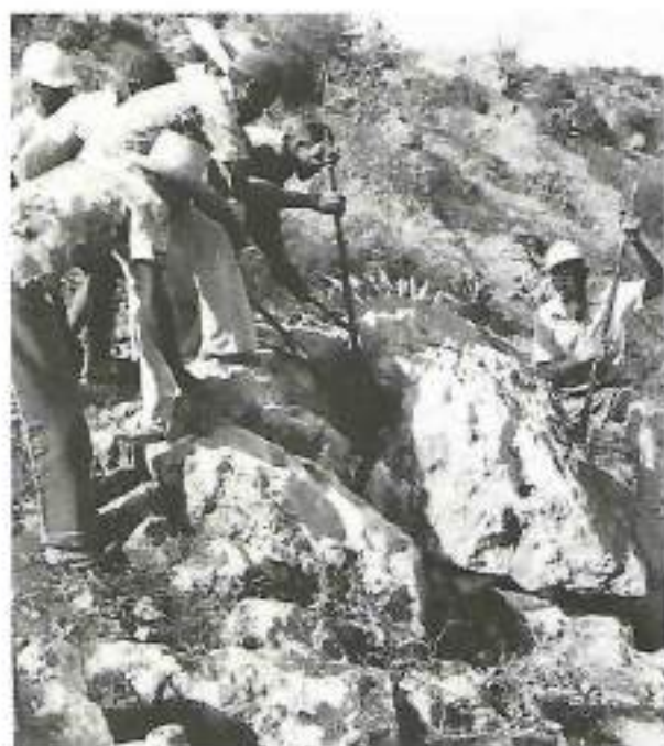
Removal of loosened blocks with quarry levers
