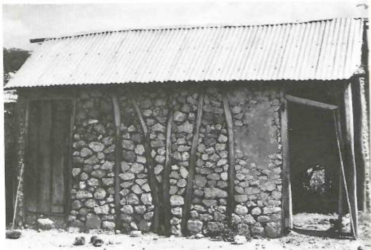
Typical rural house - Artibonite valley
