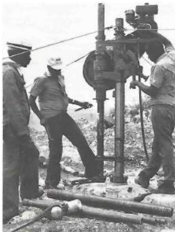
Drilling marble in La Pierre
