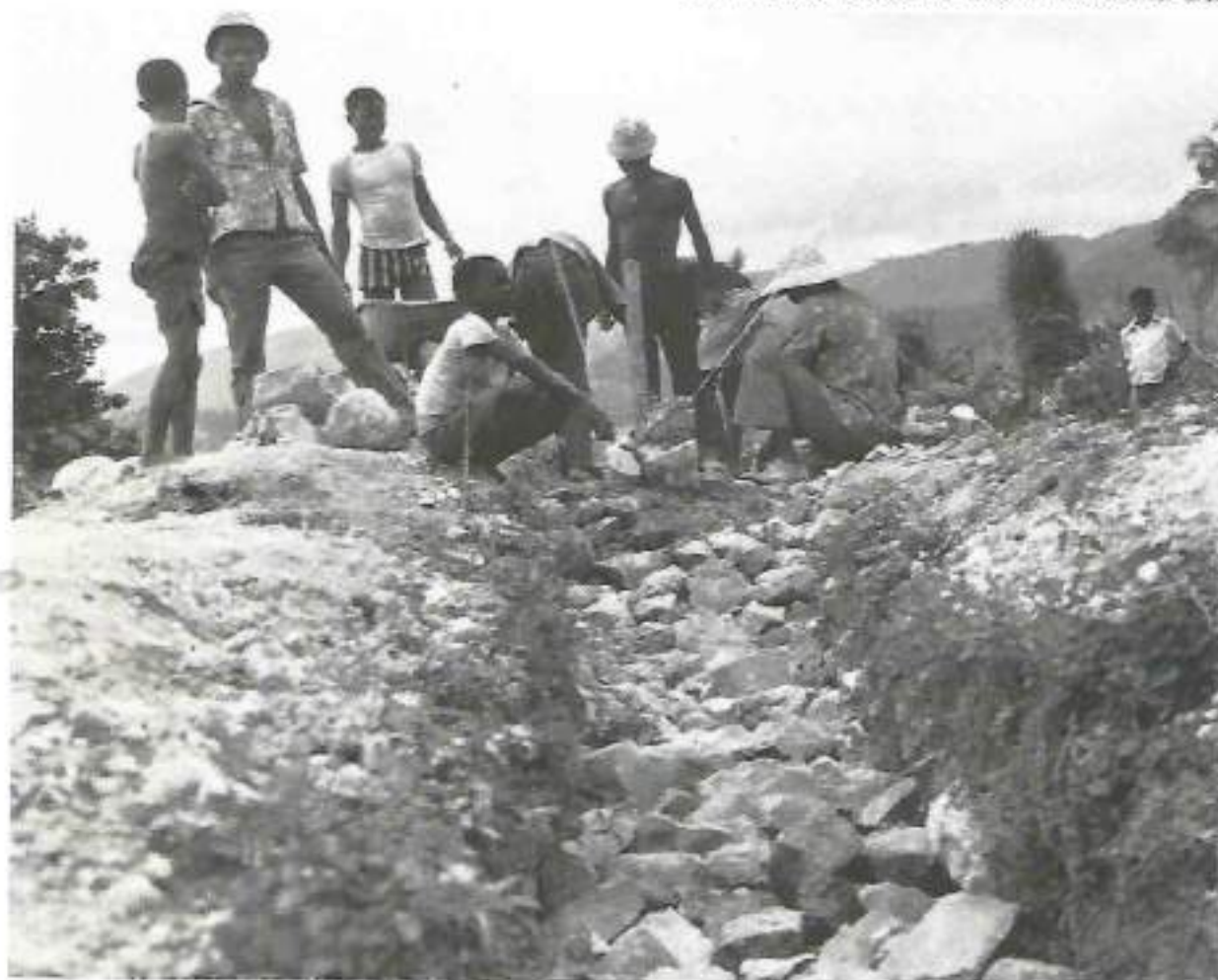
Stone foundations at Jet d'eau in the Jacmel area
