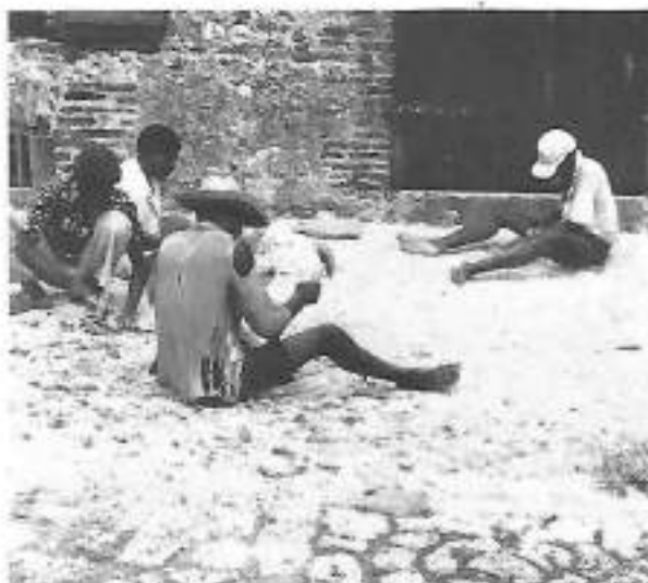
Pavement reconstruction at the Citadelle
