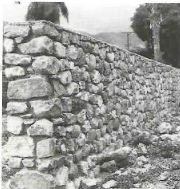
Limestone wall of undressed field stones
