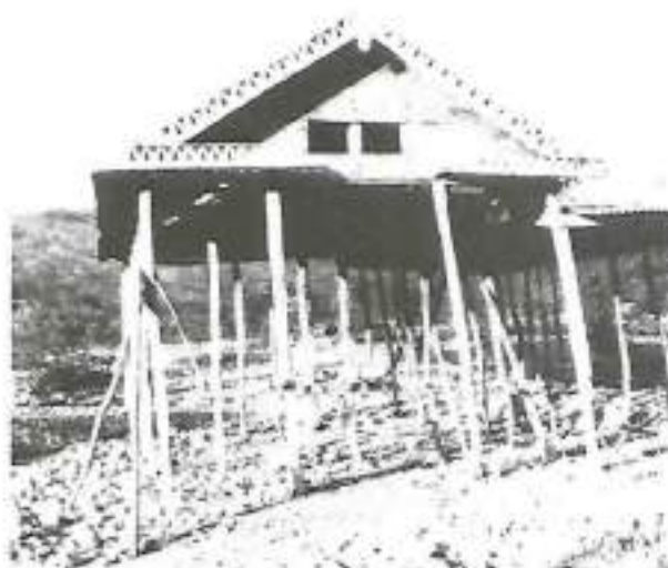
Frame ready to be filled with stone
